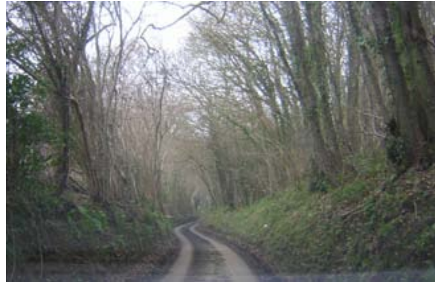
A classic holloway; the road becomes sunken over time through wear and rainwater erosion
