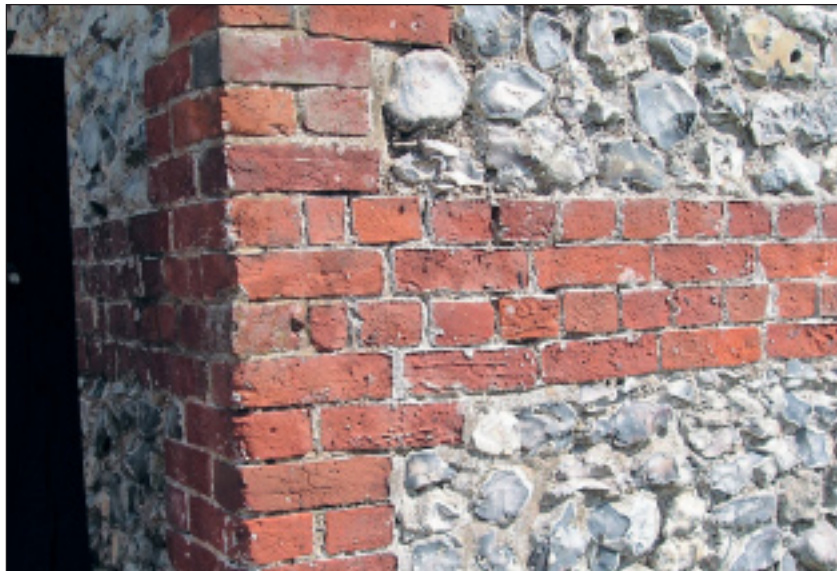
Right: Flint walling with brick quoins
